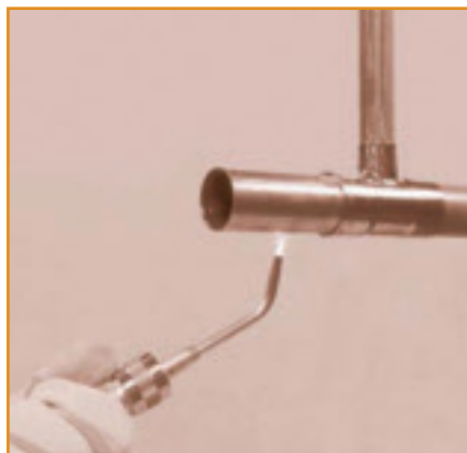
Fig. 1 — A long-standing structural application of hand soldering is in the plumbing trades. (Photo courtesy of the Copper Development Association, Inc., New York, N.Y.)
