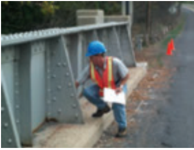
Fig. 3 — Part of a routine bridge visual inspection (Ref. 6).
