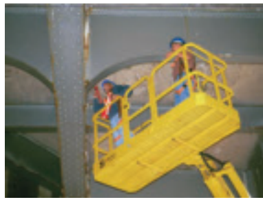
Fig. 4 — Part of an in-depth bridge visual inspection using a man-lift (Ref. 6).
