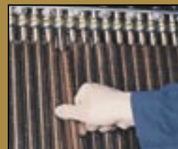
New tube is inserted into new seal. If no new tubes are available, tube holes can be plugged for tube replacement at a later date.
