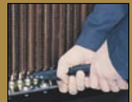
Tool seats tube into new lower seal.
