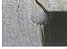
Crack propagated from angle flange after galvanizing or arising from liquid metal cracking.
