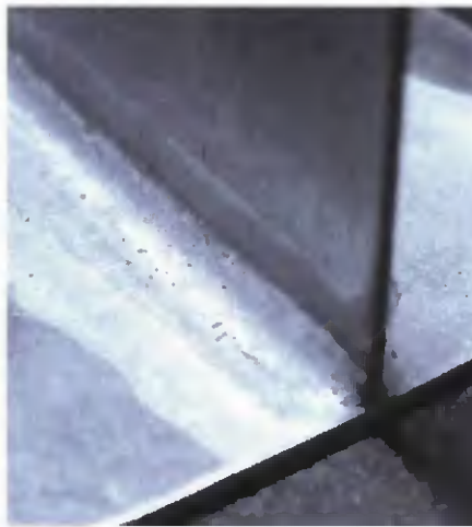
Close-up confirms good fillets on both sides. Zn-based hard solders may not be as pretty as soft solders, yet they are not susceptible to galvanic corrosion when soldering aluminum, as are Sn-based alloys.
