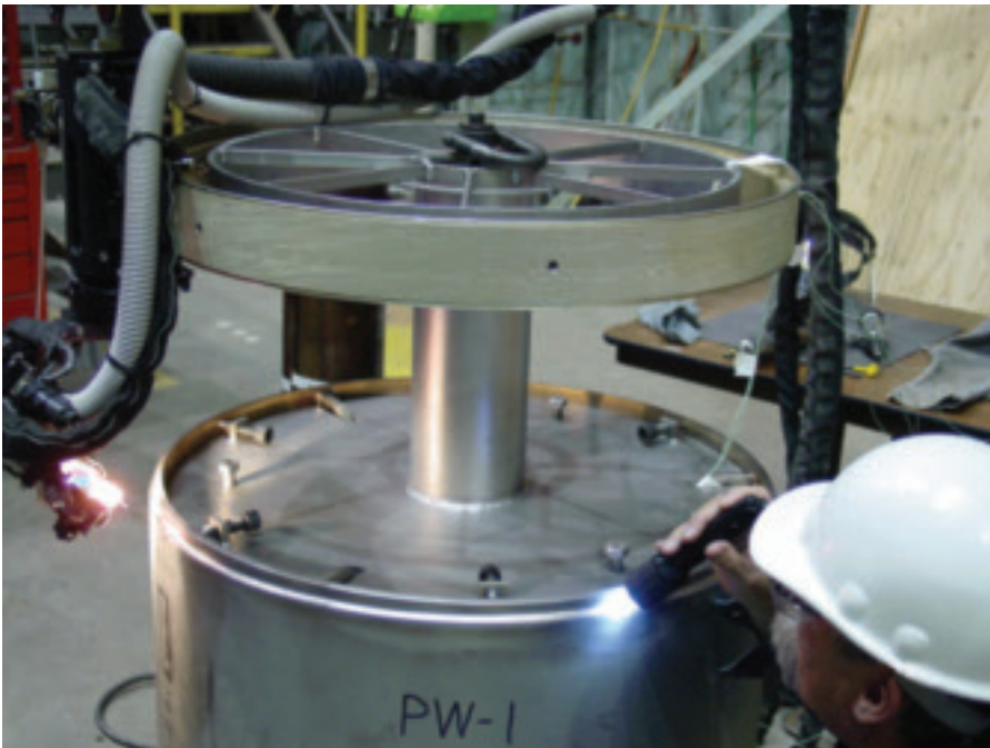
Fig. 1 — This designed and fabricated fixture supports and aligns the weld head during welding.
