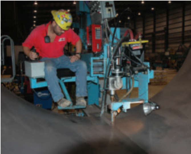
Fig. 3 — Automated SAW completes the internal welding to complete the ring.
