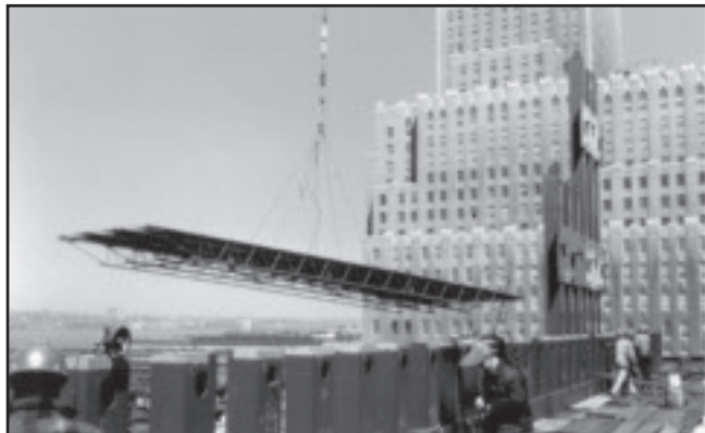
Fig. 2 — Undated construction photograph of a composite floor assembly being hoisted into place.
