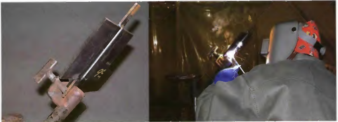
Fig. 3A — Welder qualification plate in position; B — welder training.
