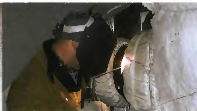
Fig. 5 — Chris Pucci deposits the first SMAW P91 root bead in North America.
