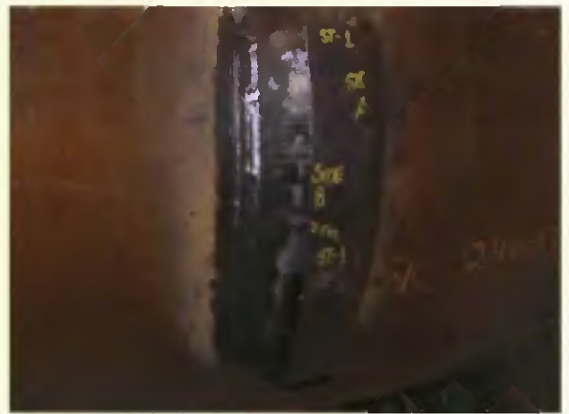
Fig. 5 — Example of completed procedure qualification trial weld.
