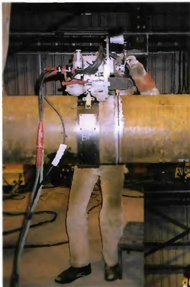
Fig. 1 — Onshore pipe-to-pipe welding using pulse gas metal arc welding.
